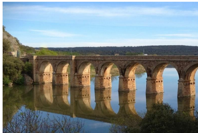
Bridge medieval over the Douro
