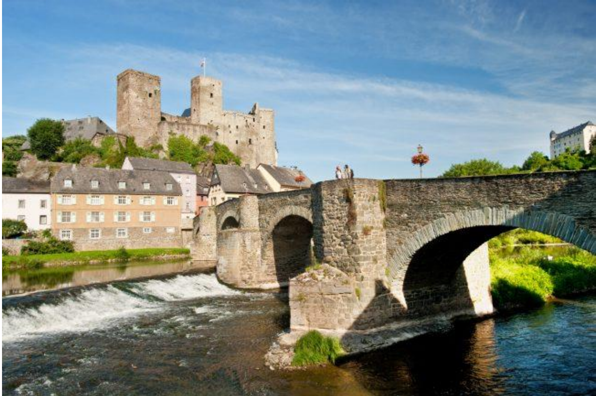
Bridge over the Lahn in Runkel
